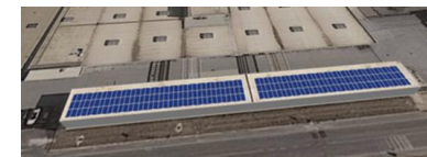
Impianto FF Blocco 10 e 11 Technosol building – 210 moduli – 114,43 kWp
